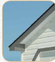
Overhang on Gable
